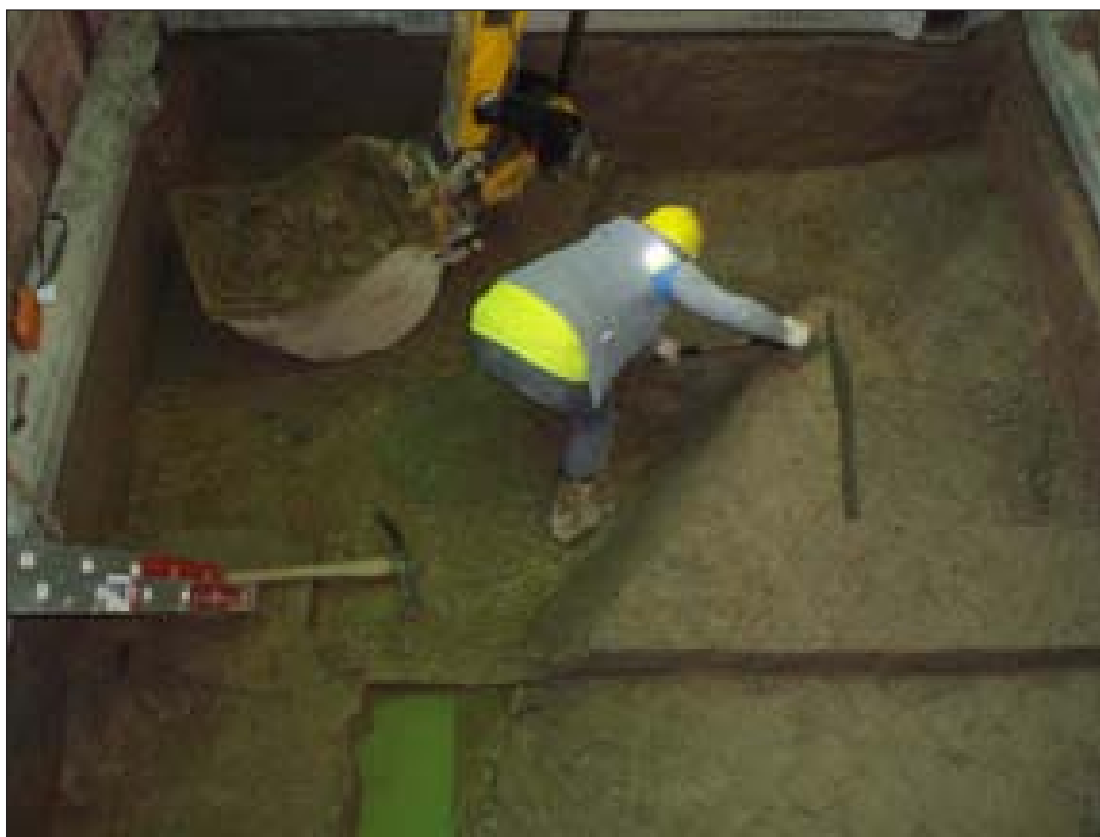
Plate 1: Trench 2, working shot
